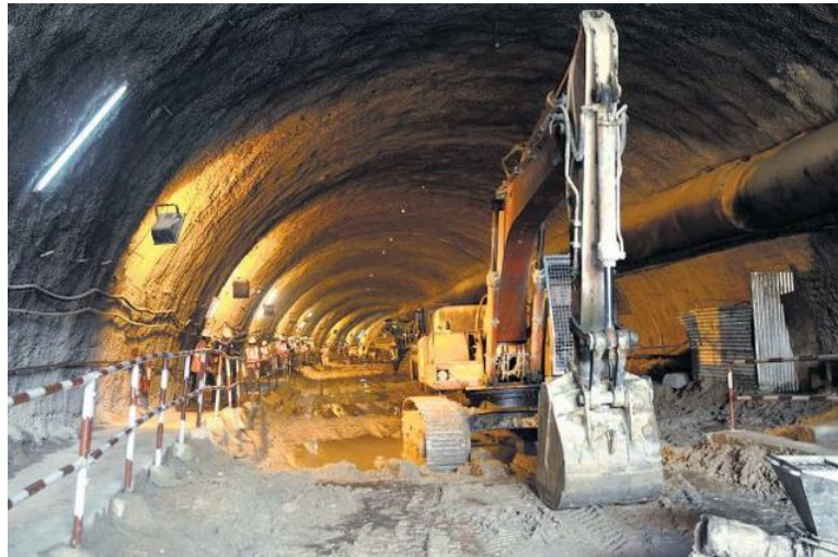
FIGURE 5.29: CONSTRUCTION OF TUNNEL BY NATM
