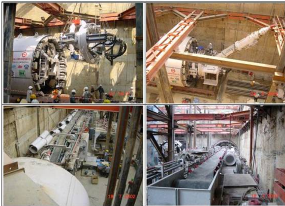
FIGURE 5.24: ERECTOR, SCREW CONVEYOR & BACKUP SYSTEM
