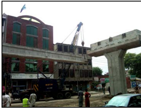
FIGURE 5.15: LAUNCHING OF I-GIRDER
