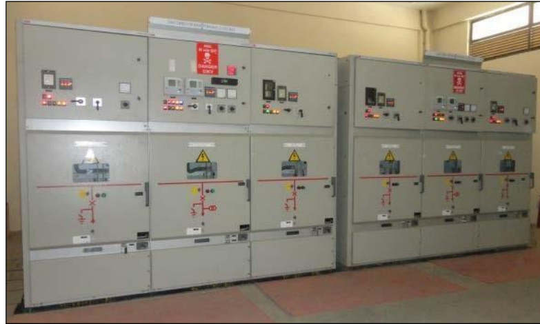
Figure 12.2: TYPICAL INDOOR AUXILIARY SUB-STATION
