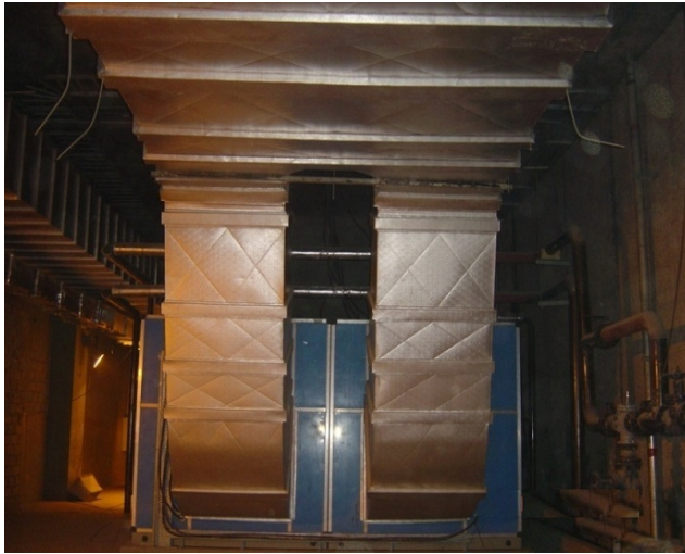
FIGURE 13.1: CONCOURSE AIR HANDLING UNIT
