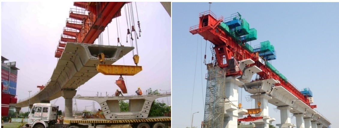
FIGURE 5.12: LAUNCHING OF BOX GIRDER SEGMENTS
