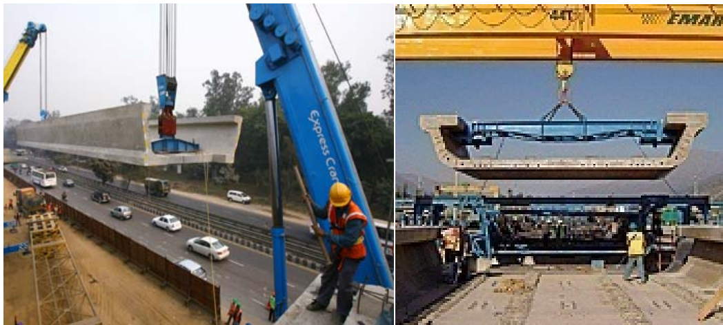
FIGURE 5.14: LAUNCHING OF U-CHANNEL GIRDER
