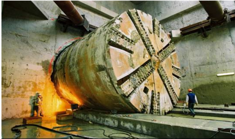
FIGURE 5.28: TBM PUSHED TO THE OTHER END OF THE STATION
