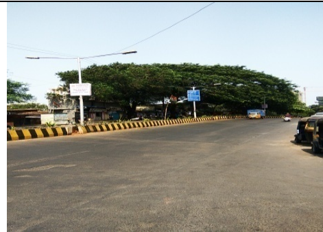
Approach road near the proposed Station
