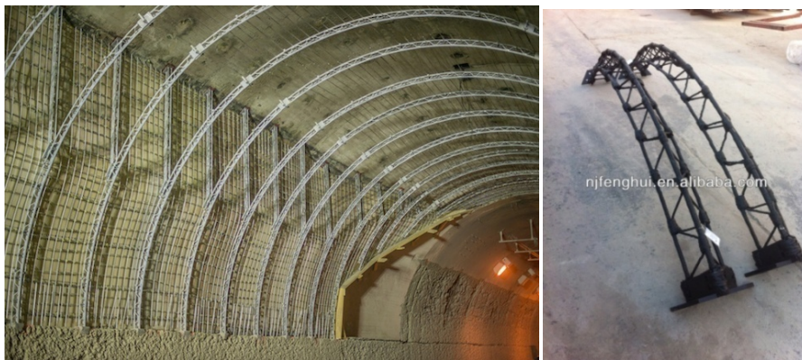
FIGURE 5.31: LATTICE GIRDER
