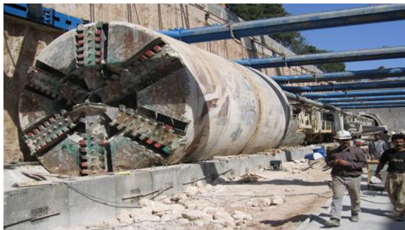
FIGURE 5.28: TBM PUSHED TO THE OTHER END OF THE STATION
