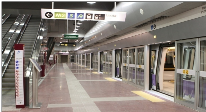
FIGURE 9.5: PLATFORM SCREEN DOOR
