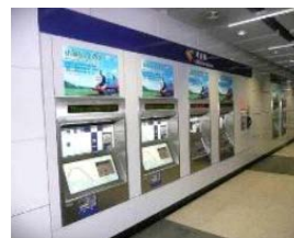
MTR Wall mounted TVM with maintenance corridor in the back – Paris
