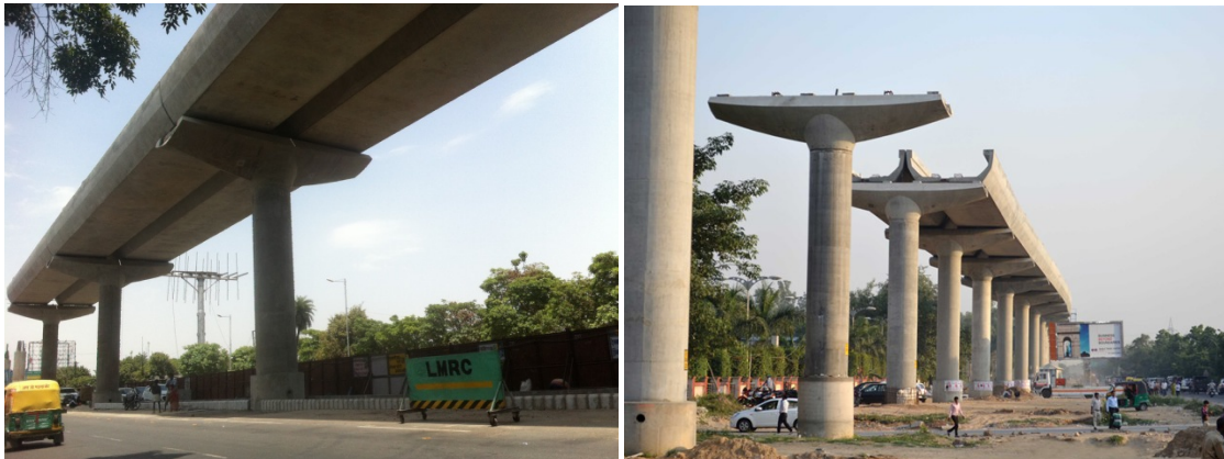
FIGURE 5.13: PRECAST U-CHANNEL SUPERSTRUCTURE
