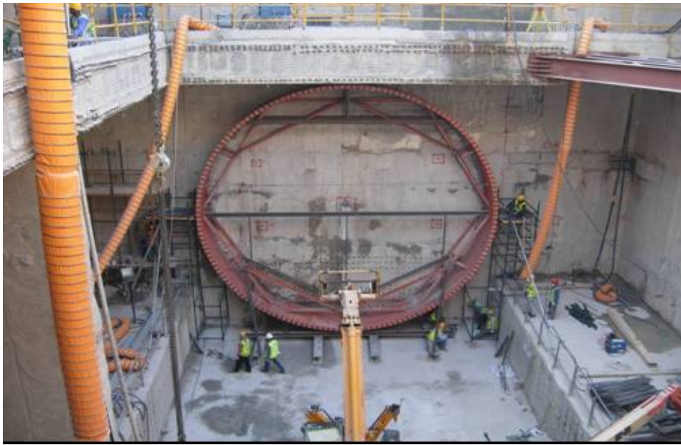
FIGURE 5.21: LAUNCHING CHAMBER
